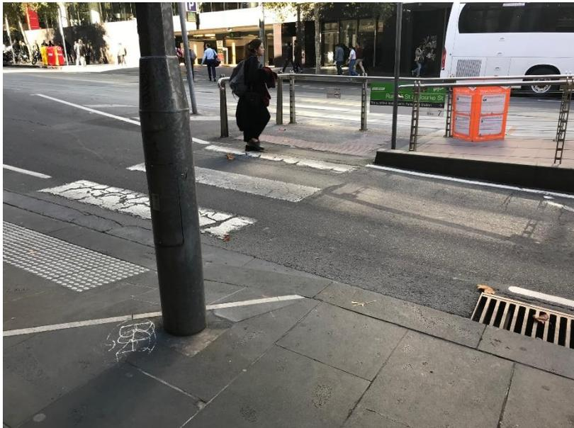
*Bourke St (north) crossing between Russell and Exhibition Streets with pram ramp extending into footpath reduces footpath width and creates potential trip hazard.*
